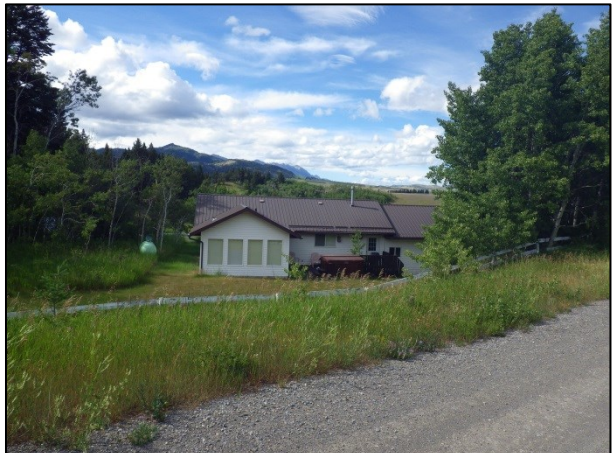
Inadequate Priority Zone 1-2 Clearance from Surface Fuels
