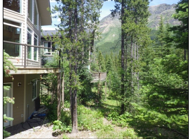
Inadequate Priority Zone 1-2 Clearance from Forest Overstory
