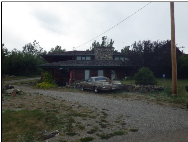
Combustible Structural Materials
